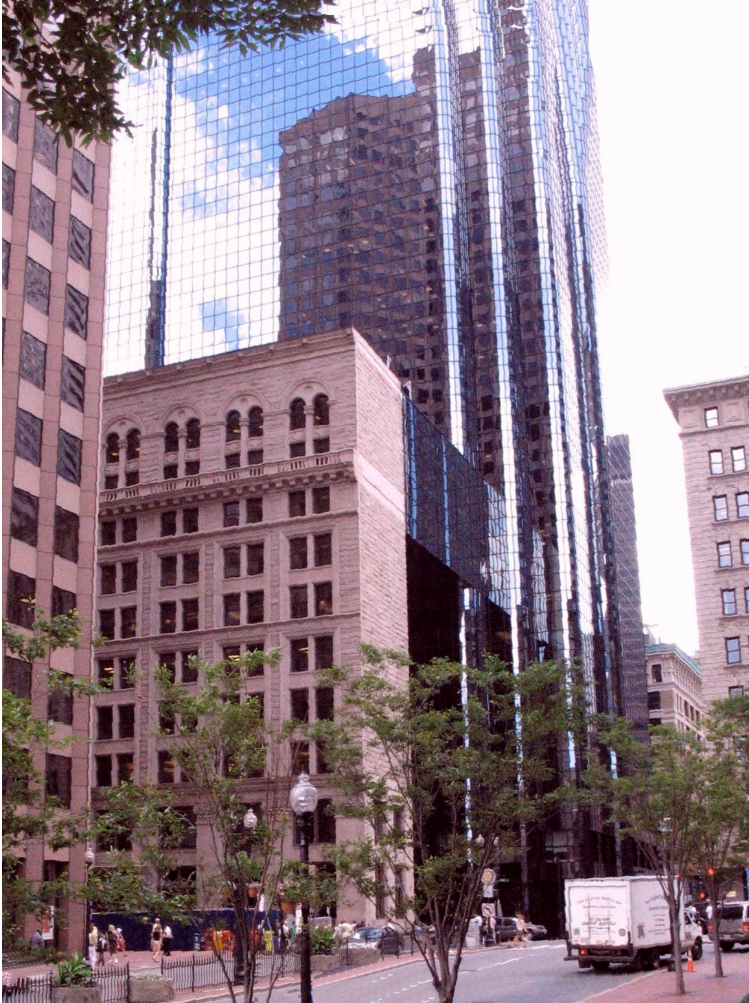
Exchange Place - 53 State Street Boston, Massachusetts
